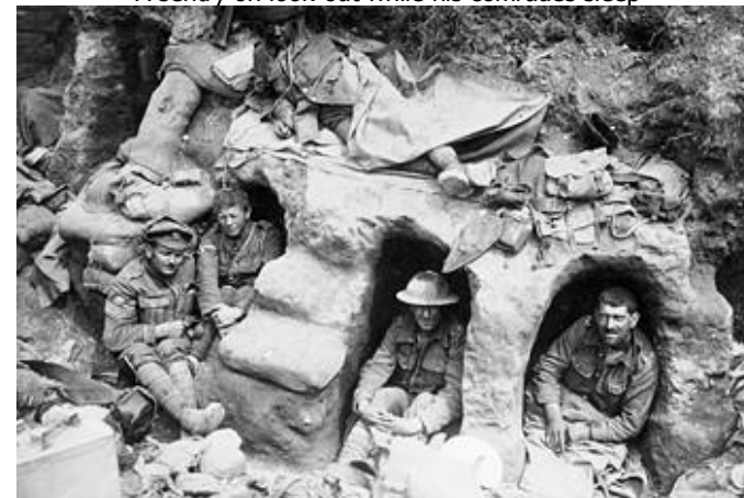
Sheltering in cubby-holes in the trench side
